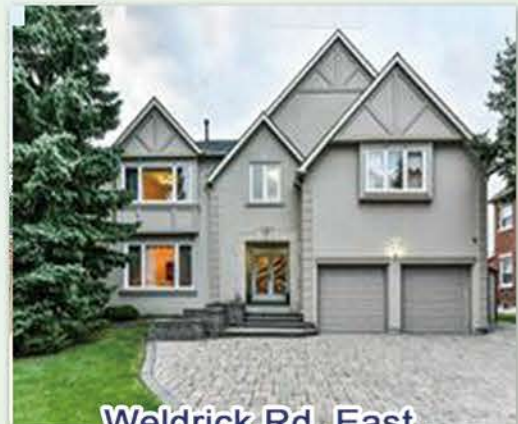
Weldrick Rd. East, Bayview Hill
