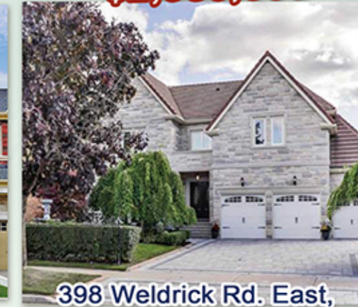
398 Weldrick Rd. East, Bayview Hill
